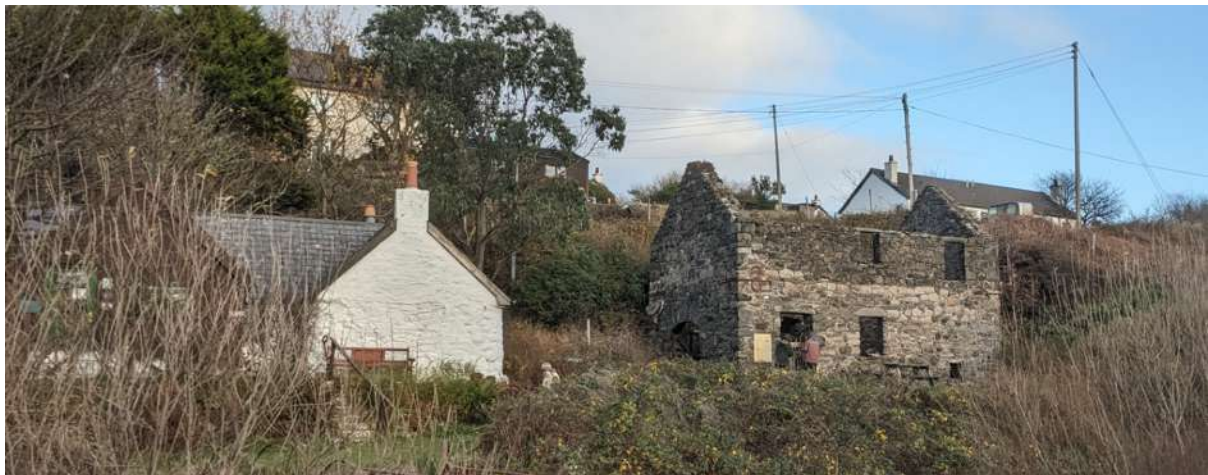
Above: the roofless Buessan Mill with Tigh na Rois, the Ross of Mull Heritage Centre in Millbrae Cottage on the left
